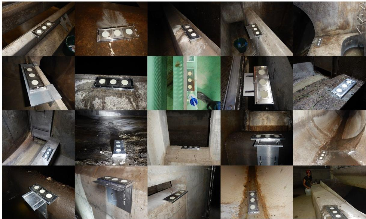
**Figure SI 1.** Installation of passive sampler mounting plates with triplicate SDB-RPS disks at the CSO (combined sewer overflow) discharge sites. The pictures are sorted by row by CSO ID.
