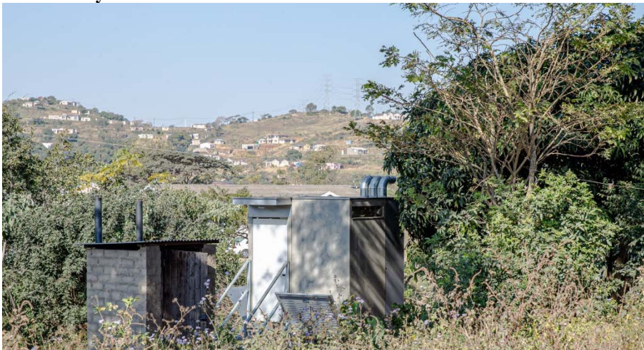
Figure S2. Photographs of the prototypes. P1 (blue) was located next to existing composting toilet facilities. P2 was installed below a shed off the main road. P3 (back) was standing behind an existing dry toilet facility.
