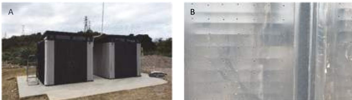
**Figure 4.17** A pilot-scale solar dryer developed by Swansea University and tested in Durban, South Africa. A) sludge is placed inside these sheds to dry. B) the walls of the sheds absorb solar energy and transfer it to the sludge inside through a ventilation system (photos: UKZN PRG).
