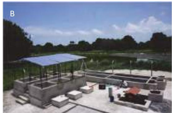
**Figure 4.9** A) mixing chitosan conditioner for pilot-scale trials. B) the pilot-scale dewatering research facility at the University of Dar es Salaam, including the settling-thickening tanks, conditioner mixing tank, and six sand drying beds (photos: Eawag).
