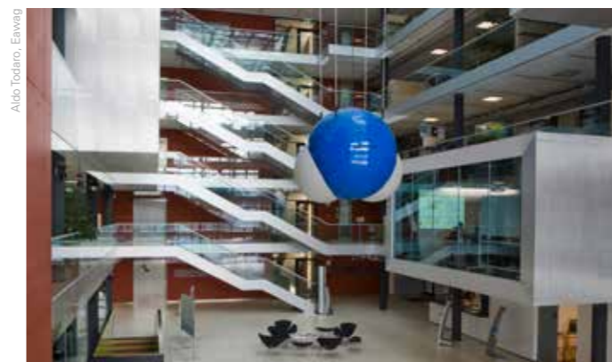
Forum Chriesbach, Eawag's main building, is one of the world's greenest buildings.
