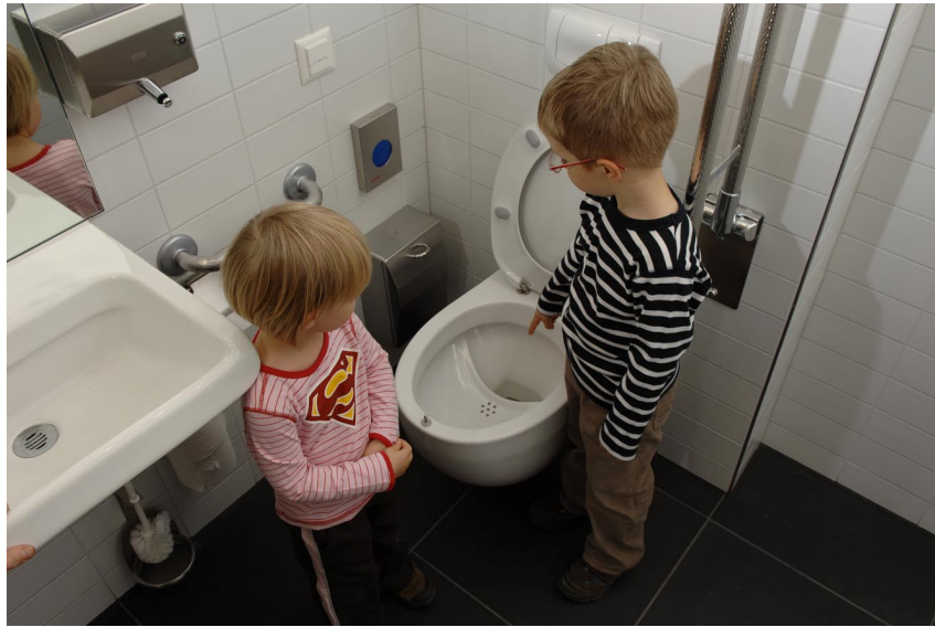
Figure 3. How does a NoMix toilet work? NoMix toilets allow separate collection of urine, which can be stored in a tank in the cellar. The urine is drained off in the front bowl; the rest reaches the sewers as in any toilet. In principle, NoMix toilets can be used like conventional toilets – if one sits to urinate. However, especially children may have problems with the proper sitting position. This model is by Roediger ( www.roevac.com ). Photo: Ruedi Keller, 2006.
