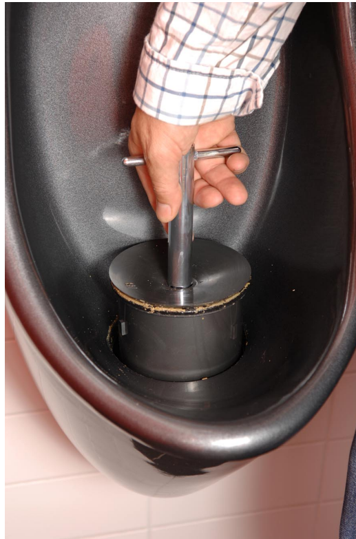
Figure 4. Removal of precipitates in waterfree urinals. All NoMix installations need very good cleaning and maintenance. Some waterfree urinals require regular exchange of the stench trap. Future developments of NoMix toilets by the sanitary industry could involve a similar solution: Controlled precipitation of struvite could be provoked in the NoMix toilets. This would not only minimize blockages, but could be an elegant way to recover phosphorus for fertilizer use. This urinal is by Hellbrok ( www.hellbrok.com ). Photo: Ruedi Keller, 2006.
