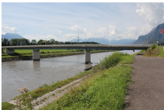
Figure 9: Bridge over the river Rhine near Oberriet in Switzerland.
