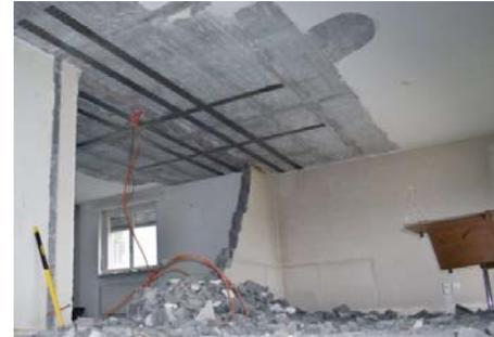
Figure 9. Multi-story building in Goldach (CH): Strengthening of RC slabs over 14 stories due to new openings (left), Residential building in Brunnen (CH): Strengthening of RC slabs due to removal of load-carrying walls, a total of 12 re-plates was installed (right)
