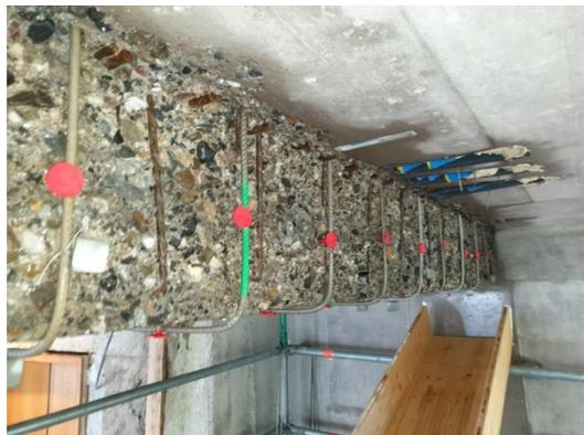
Figure 12. U-shaped re-bars for prestressed shear strengthening. Sprayed mortar will be used subsequently to embed the bars prior to activation by
