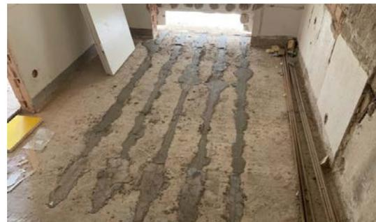
Figure 11. Activation of end-anchored re-bars with infrared heating units (left), RC slab, strengthened with near-surface mounted re-bars (right)
