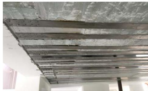
Figure 7. Residential building, Hinwil (CH): Strengthening of cantilever RC slab with 5 m span against deformation due to negative bending moment, 18 re-plates with lengths up to 7 m were used (left), Residential building, Zumikon (CH): Combined use of re-plate and CFRP strips for strengthening of RC slab, installation of 14 re-plates (right)
