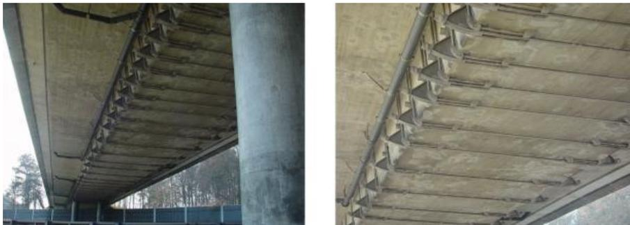
Figure 3: Bridge over the Swiss motorway A1 with shear strengthening.
