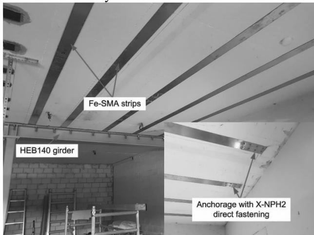
Figure 1 Re-plates (Fe-SMA strips) are installed as pre-stressed strengthening elements for a reinforced concrete slab [Michels et al. (2018)]
