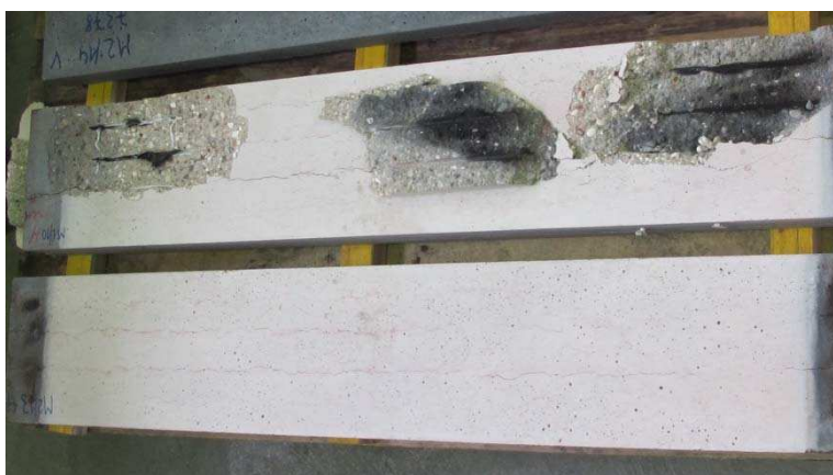
Figure 5. Fire exposed surface of specimen 1_Ref after 90 minutes in the fire denoting 3 spalled areas (above), next to specimen 3_SAP without spalling (below, tested in the same fire experiment as 1_Ref).
