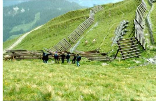
Fig. 3: Snow supporting structures destroyed by an avalanche, which was released high above the controlled area. The structural safety is not fulfilled for impacts of large avalanches. The reliability is low.
