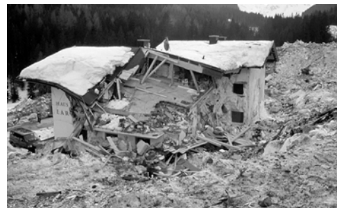
Figure 1: Photo of a house damaged by a snow avalanche in Valzur near Galtür, Austria, 1999, S. Margreth photo.
